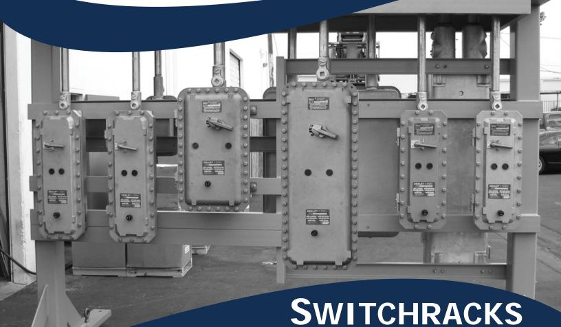
Equipment Racks with NEMA 4/4X and NEMA 7/9 Explosionproof Classified Enclosures
